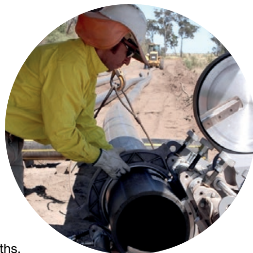
Figure 3. Typical butt welding machine used for PE pipe joining.
