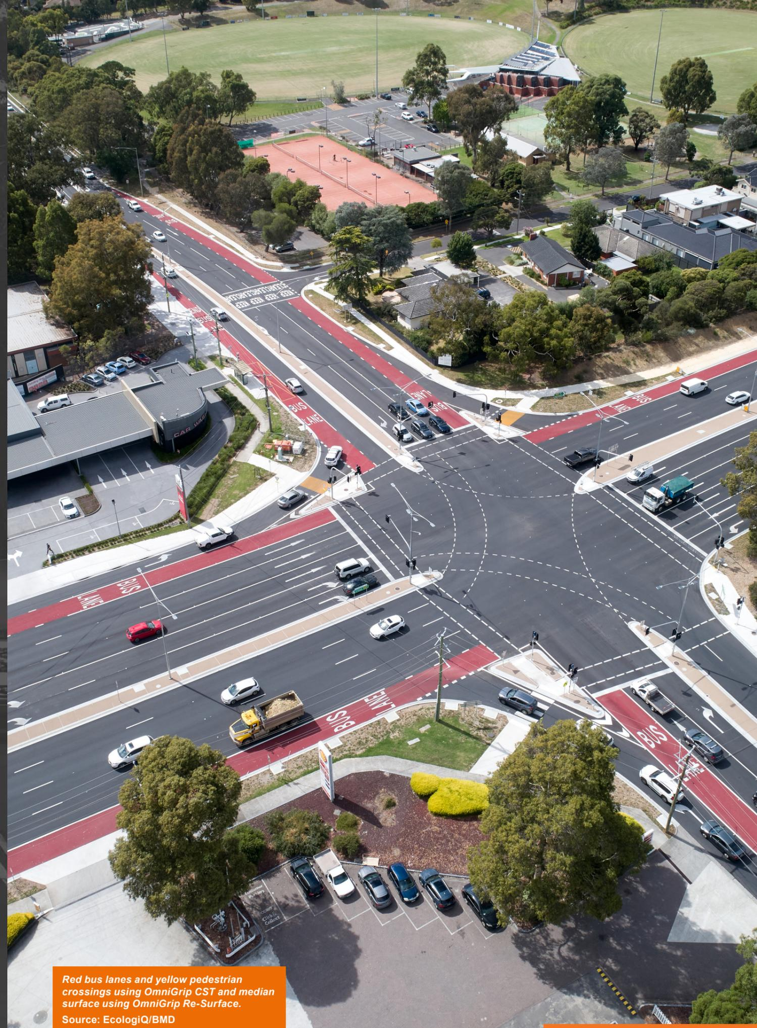
Red bus lanes and yellow pedestrian crossings using OmniGrip CST and median surface using OmniGrip Re-Surface.
