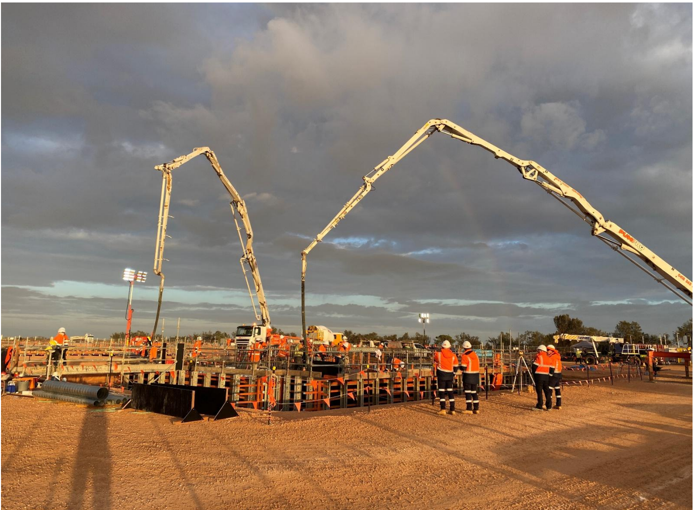
Photo above: (Buronga Substation – Large Synchon pour, 850m 3 )
