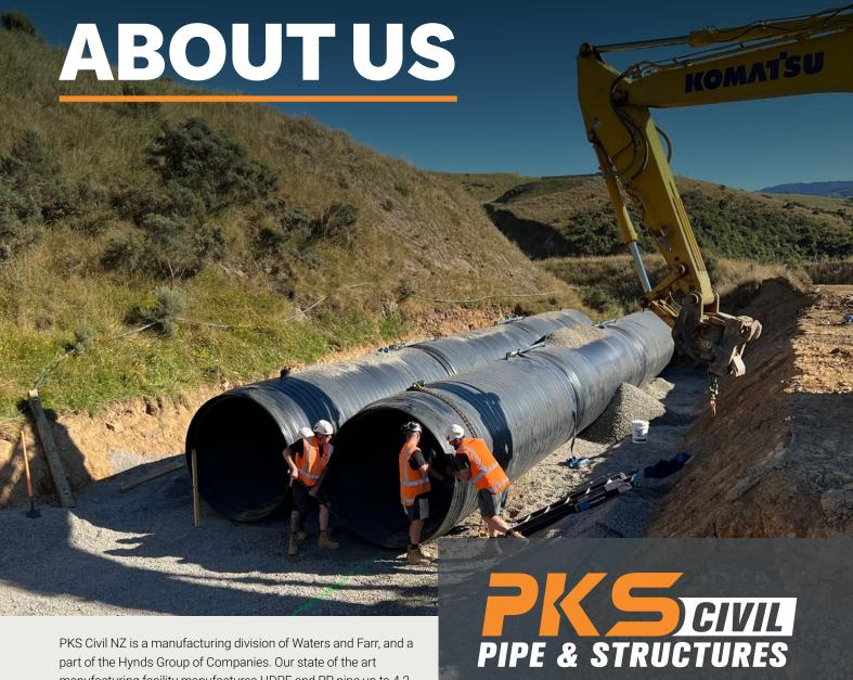
manufacturing facility manufactures HDPE and PP pipe up to 4.2 m in diameter (project specific), along with manhole and pipeline structures for water storage, wet wells and intake manifold needs.
